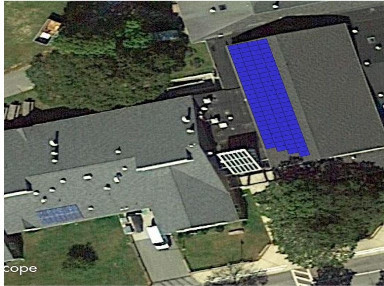
Figure 4. Solar PV Siting at the School
